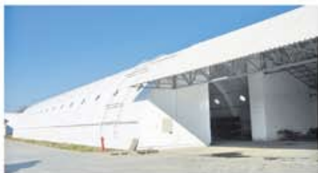
2008, Boljevci Production hall 17x56m
