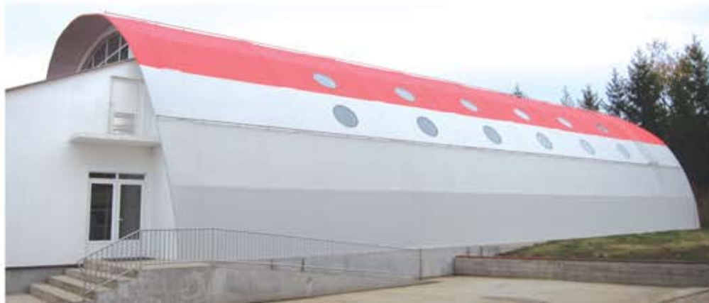
2011, Stalać (Čičevac) School sports hall, 17x32m
